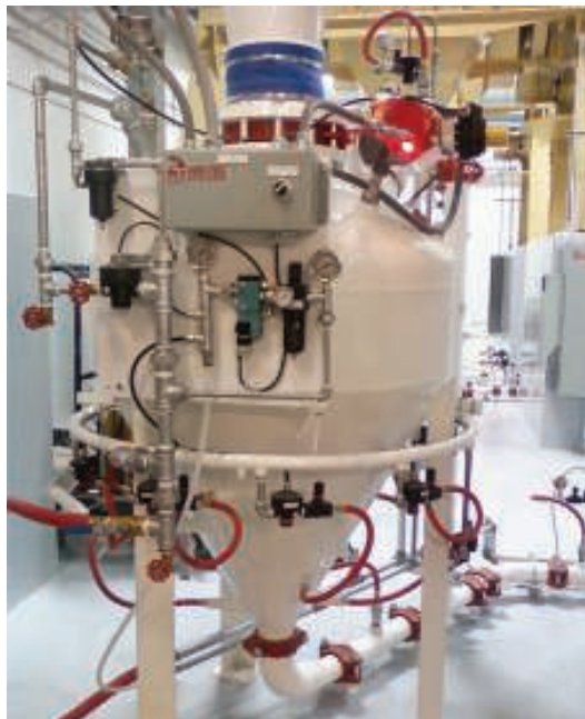
FIGURE 1. To overcome resistance in the conveying line, NoI-Tec Air Assits are placed strategically to distribute energy throughout the transport system. This results in increased efficiency and reliability
