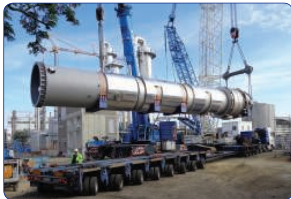
GEA's innovative column design uses multiple vapor-recompression units to slash energy requirements
