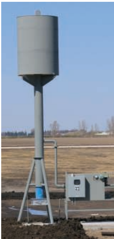
FIGURE 8. Shown here (above left and top) is a small, elevated enclosed flare that operates in a “smokeless,” air-assisted type
