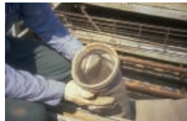
FIGURE 2. The image at left shows two baghouses installed in parallel. On the right, the cage is inserted into filter bags, and pulse-jet pipes provide blowback to clean the dust off the filter
