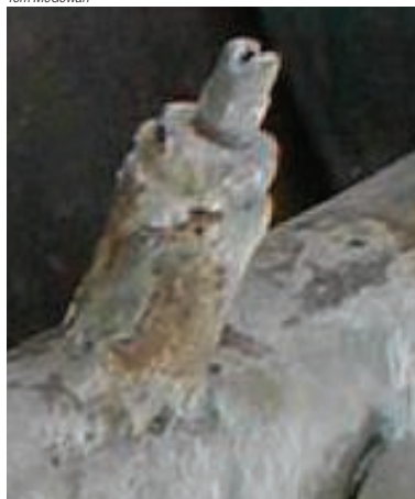
FIGURE 6. Fouling of spray nozzle by lime solids requires periodic changeout or chemical treatment
